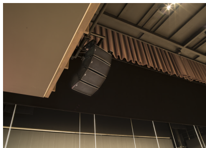
The main speakers at the Kani Public Arts Center small theater are NEXO GEO M6 units
